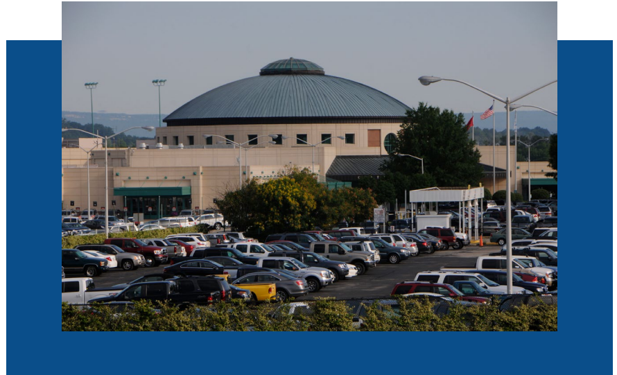
Shown: The Chattanooga Airport roof prior to the storm in 2019
